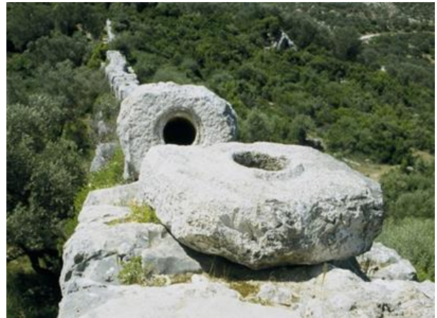
The Siphon – It was sealed with molten Lead
